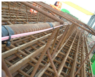
Cable glued inside a penstock
