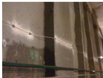
Cable clamped on concrete blocks
