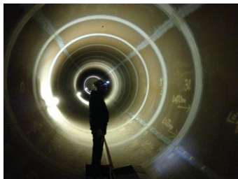
Cable glued inside a penstock
