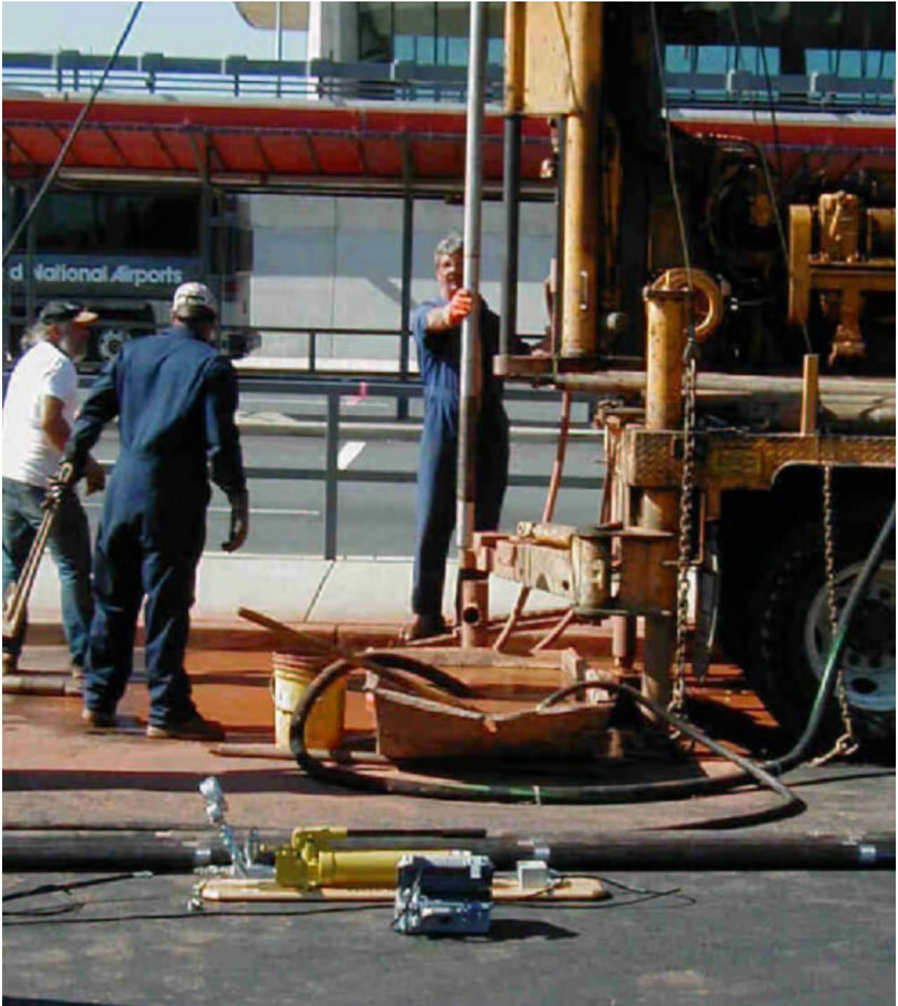
Photo 1. Rock pressuremeter being lowered into borehole
