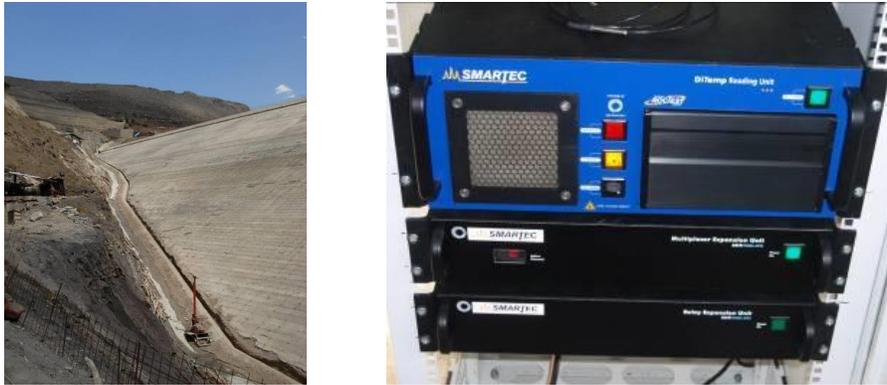
Fig. 5 Sensing cable installation at the plinth of the upstream face of the upper dam and one monitoring cabinet
