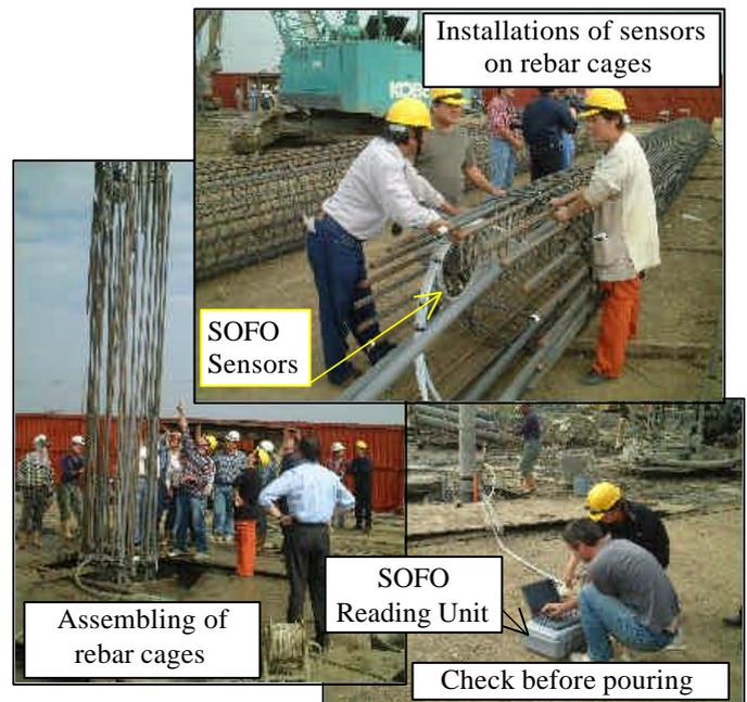
Figure 6: Installation of SOFO sensors on rebar cages.
