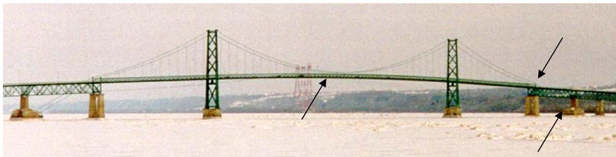
Figure 1. Side view of the Île-d'Orléans bridge (arrows point to locations where the main cable was opened and the anchor block was tested).
