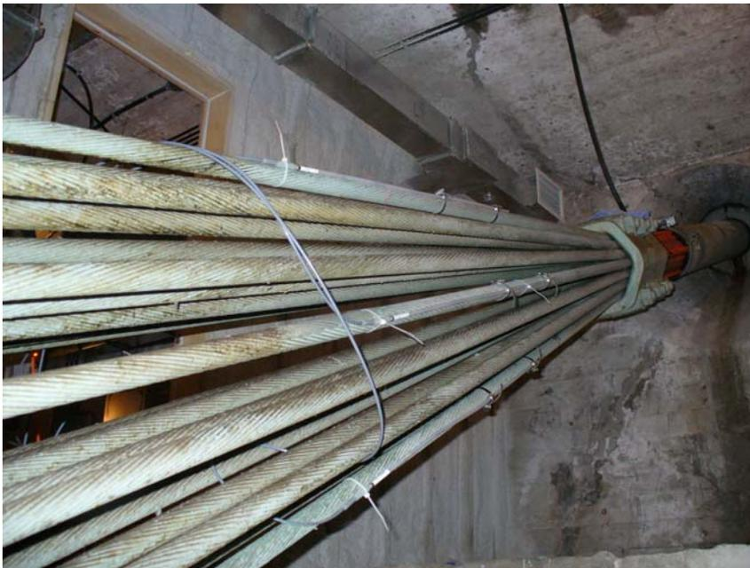
Figure 5. SOFO sensors, cable section in the anchorage chamber.
