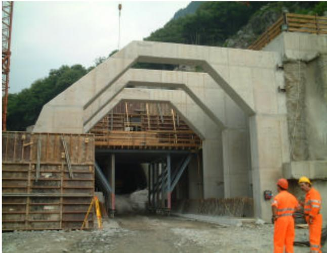
Figure 8: Support Butresses at the south portal of the new Alptransit Gotthard tunnel
