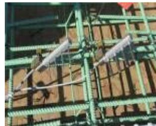
Concrete humidity and corrosion sensors
