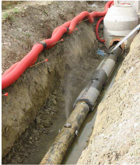
Fig. 10. Test pipe before DTS cable installation. Fig.11. DTS cables support cage placed over the test pipe.
