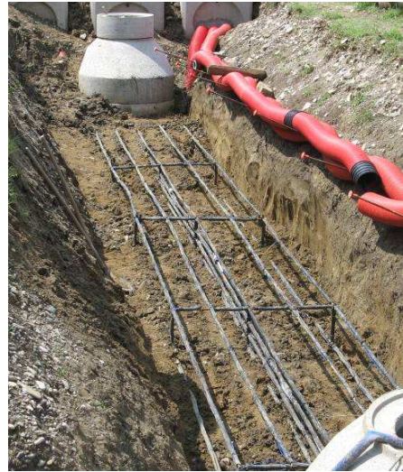
Fig. 10. Test pipe before DTS cable installation. Fig.11. DTS cables support cage placed over the test pipe.
