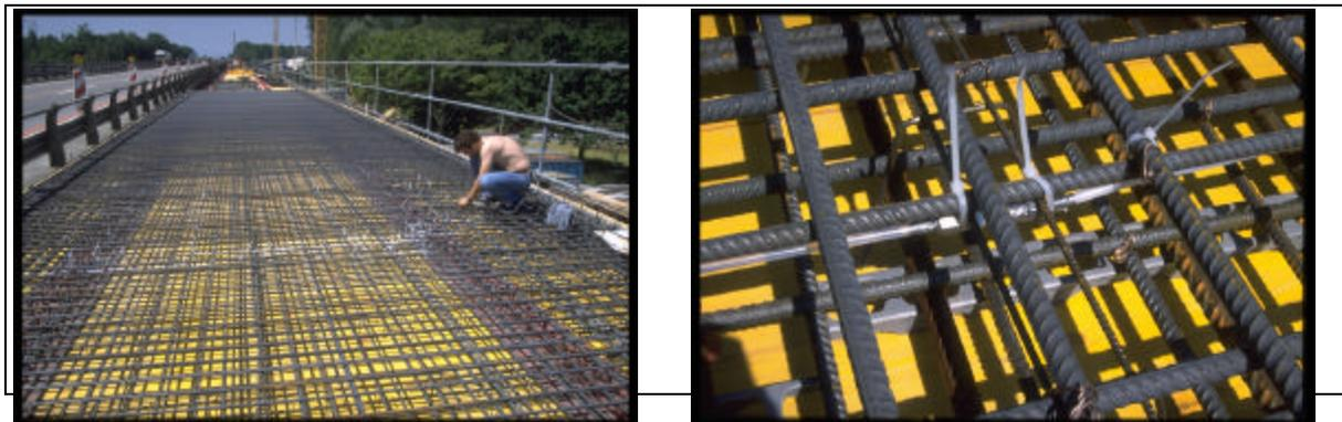
*Figure 5 a) General view of the section 1. b) Fixation of the sensor to the framework
