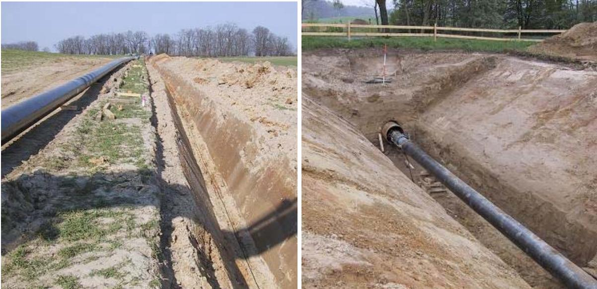
*Fig. 5 : Construction phase of a buried brine pipeline in the north-east area of Berlin. The fiber optics cable is placed in the sand at the 6 o'clock position about 10 cm underneath the pipeline .*
