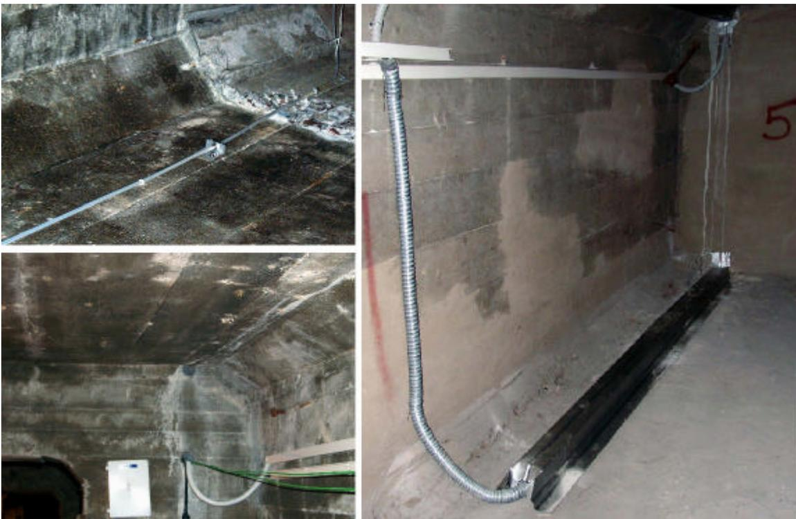
Figure 3: Bolshoi Moskvoretskiy Bridge: SOFO sensor before and after the protection is installed, and a view to the intermediate connection box. Courtesy of Triada Holding, Moscow
