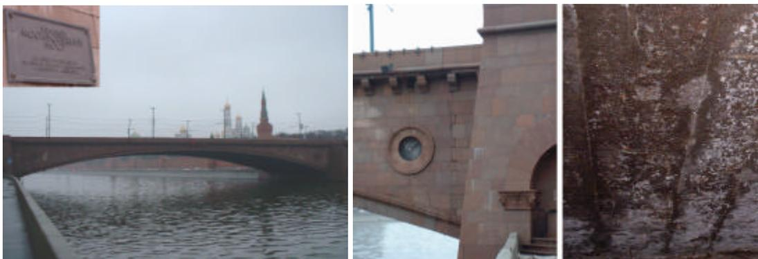
Figure 1: Bolshoi Moskvoretskiy Bridge: general view, cracking of the stone walls confirms the settlement in the middle of the arch; penetration of chlorides is visible in the interior of the arch boxes. Courtesy of Triada Holding, Moscow
