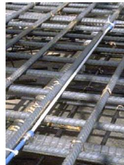
Figure 2: SOFO Sensor installed on a rebar
