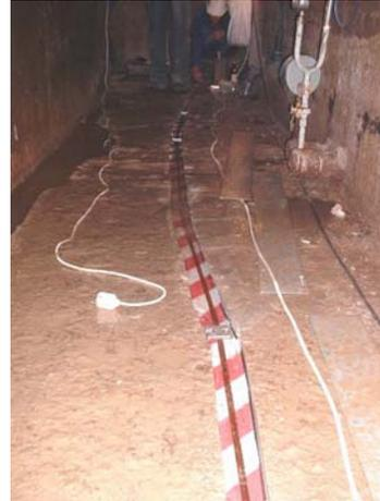
Figure 12: SMARTape installation in the inspection gallery.
