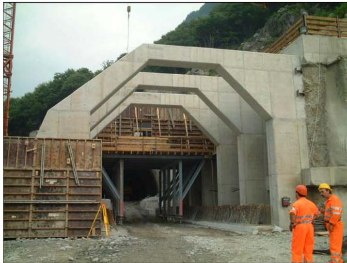
Figure 8: Support Buttresses at the south portal of the new Alptransit Gotthard tunnel
