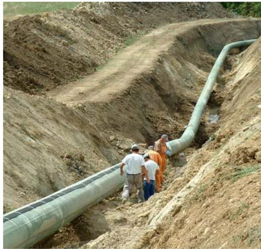
Figure 9: SMARTape on the gas pipeline.
