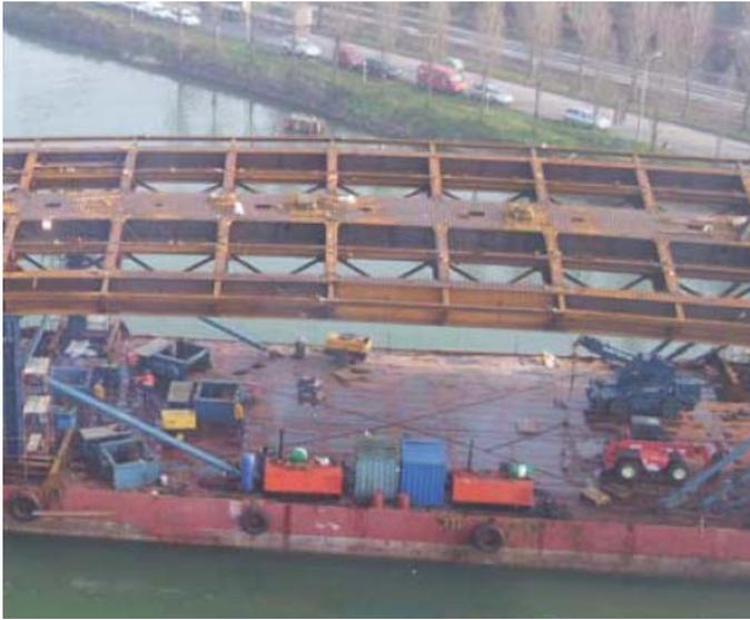
Figure 2 – View of the steel deck during transport
