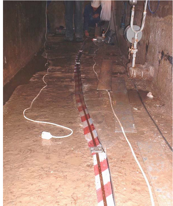
Figure 7: SMARTape installation in the inspection gallery.
