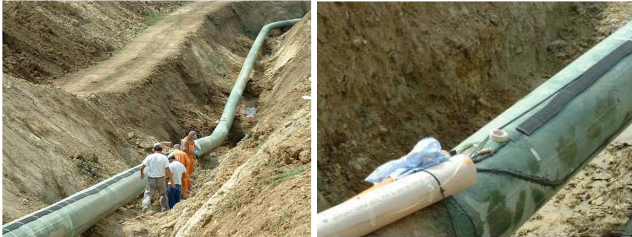
Figure 8: SMARTape on the gas pipeline.
