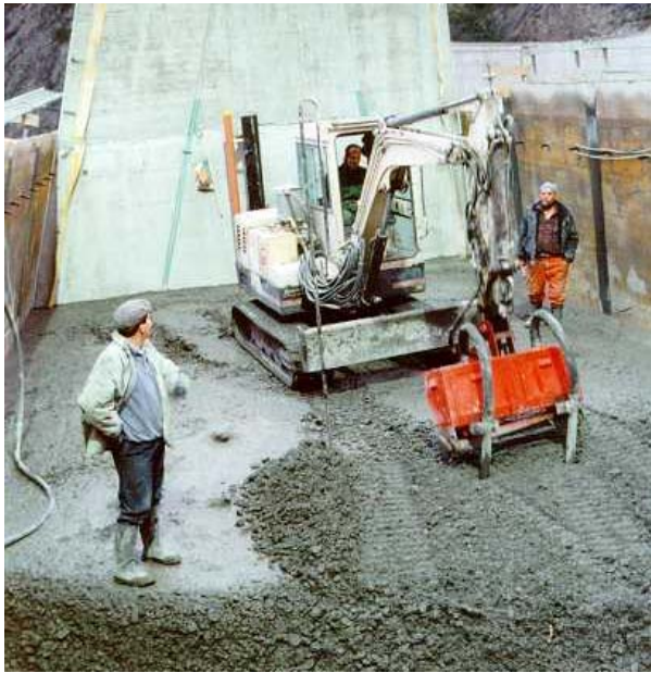
Figure 4: Luzzone Dam raising works
