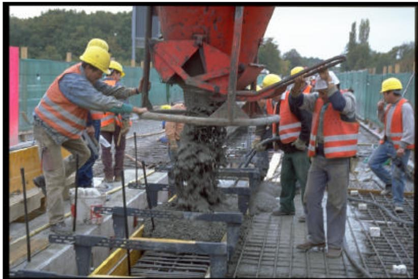
*Figure 8: The concrete was poured on the sensors without any precaution*
