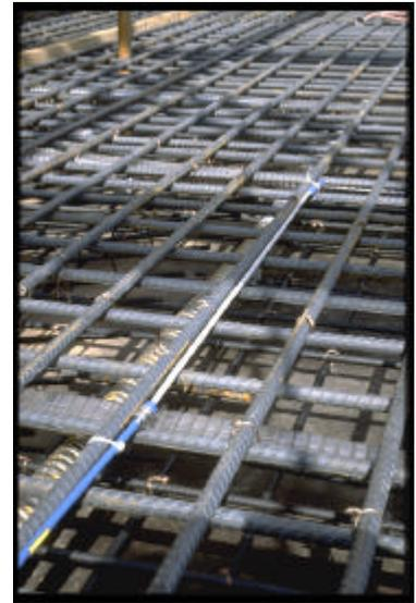
*Figure 7: Fixation of the sensor to the framework. Sensor are held but not fixed to the re bars with plastic ring*
