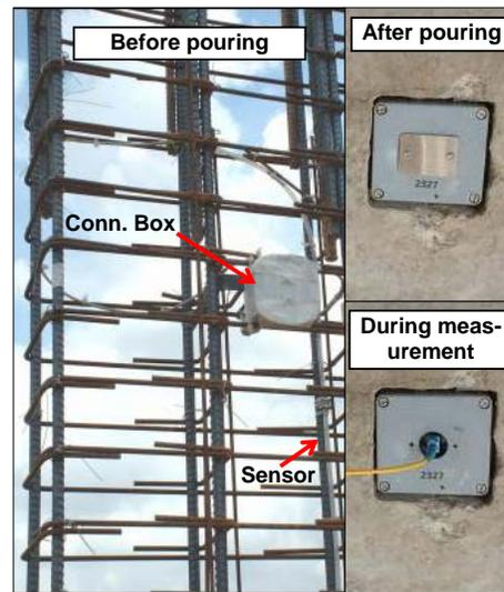
Figure 3. Sensor and connection box installed on a rebar cage, and connection box after the pouring of columns
