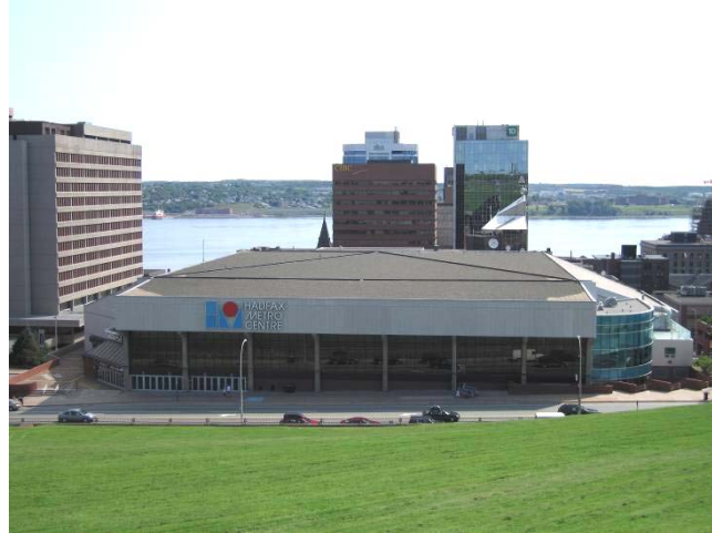
Figure 12: The Metro Centre arena in Halifax
