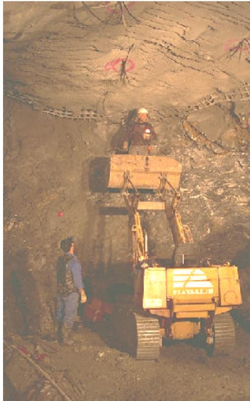
Figure 4.2: Installation of the SOFO sensors in section 1.
