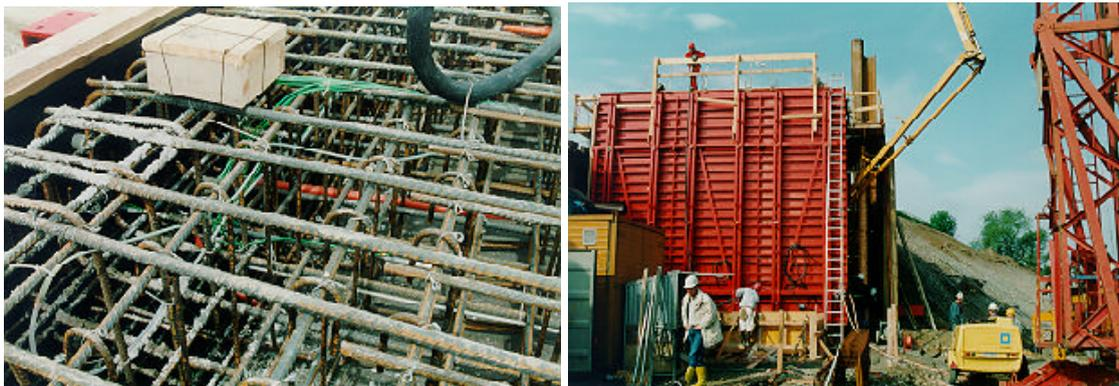
Figure 4.3: Sensor installation and concrete pouring at the N5 tunnel.
