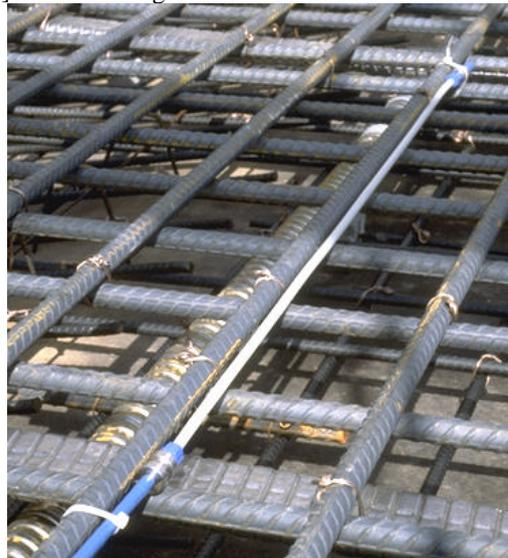
Figure 4 SOFO sensor installed along a rebar before concreting.
