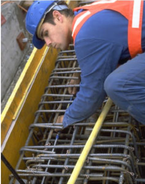
**Figure 7: Sensor installation in concrete**
