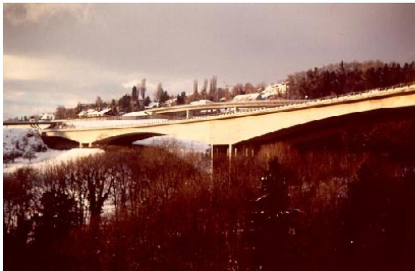
section. It consists of a box girder of variable height (from 2.5m to 8.5m) and two slightly asymmetric cantilevers meant to reduce the effect of torsion in the curved bridges.
