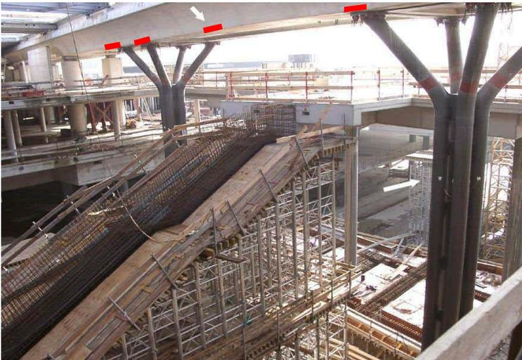
Fig. 1: Two fork columns in the central part of the southern railway bridge
