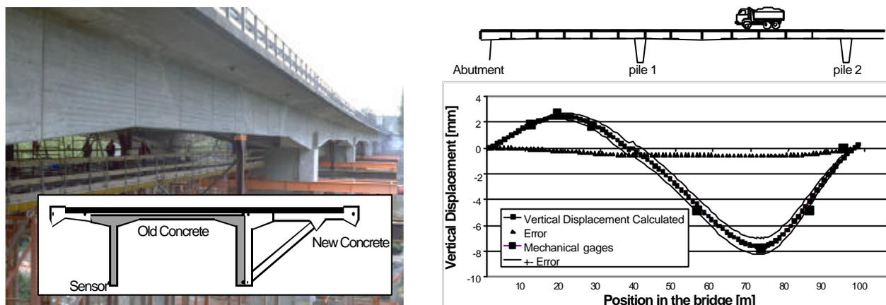
Fig. 3: Versoix Bridge, general view and sensor placement in a typical cross-section (left); vertical displacements calculated from SOFO curvature measurements compared with wire extensometers readings (Courtesy of S. Vurpillot, IMAC-EPFL, Switzerland) (right)
