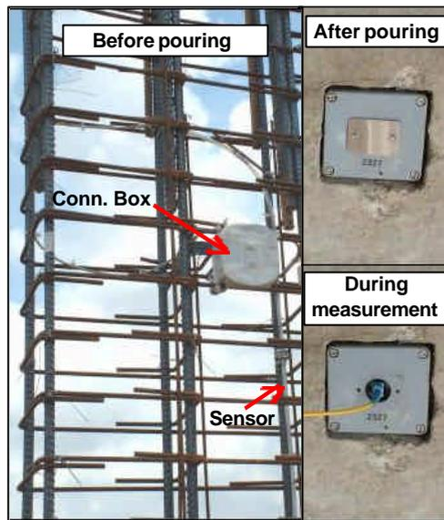
Fig. 4: Sensor and connection box installed on a rebar cage, and connection box after the pouring of columns
