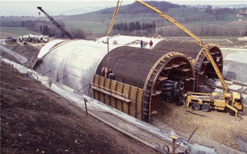
Figure 3: Champ Baly Cut-and-cover Tunnel under Construction
