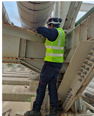
Fiber optic leak detection sensing cable installation on ammonia pipelines
