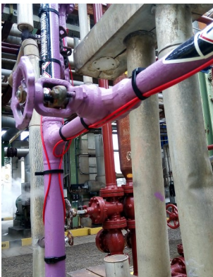
Fiber optic leak detection sensing cable installation on ammonia pipelines
