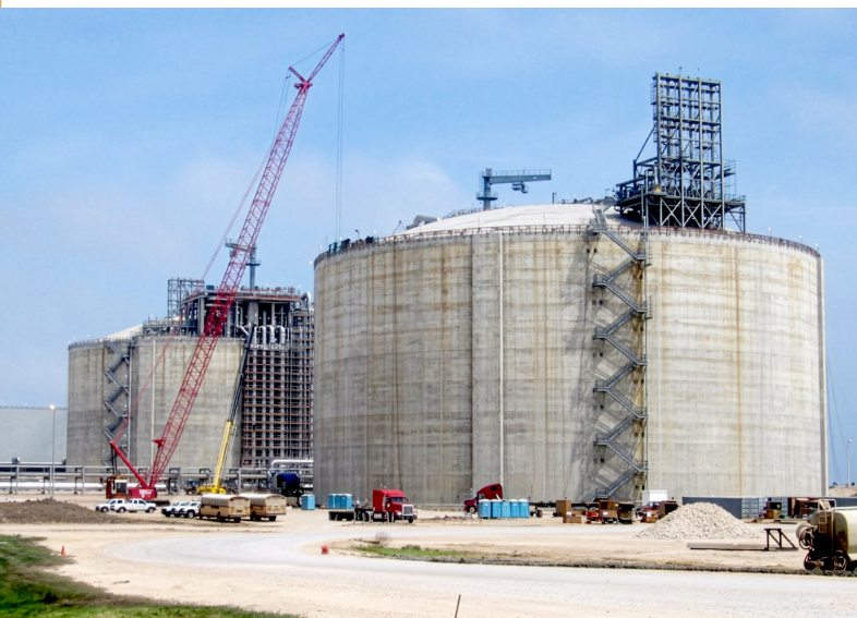
Construction at the LNG storage tanks in Thailand at the Nong Fab LNG Receiving Terminal in Rayong.
