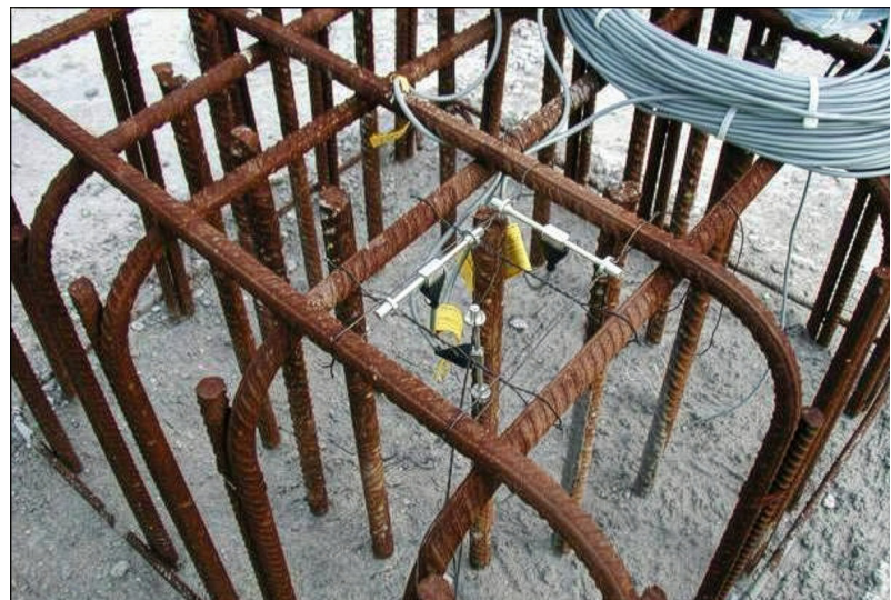
Strain gauges and temperature sensors being installed during construction.
