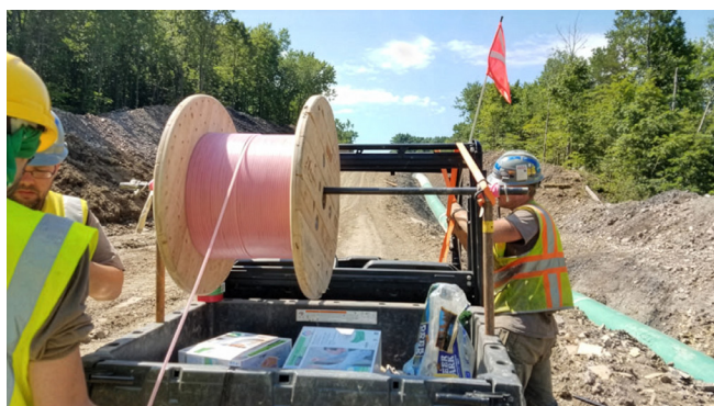
Strain sensing cable on spool before installation
